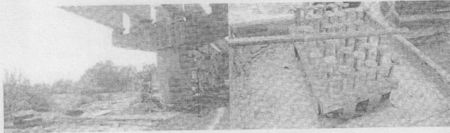
Figure 4 :Close View of Temporary wooden Bearing, Pier and Pier cap/beam near Railway Line and Sharp edges of concrete and bearing Pedestal without cracking. Railway line is farther just after green grass/trees shown in the Figure.
