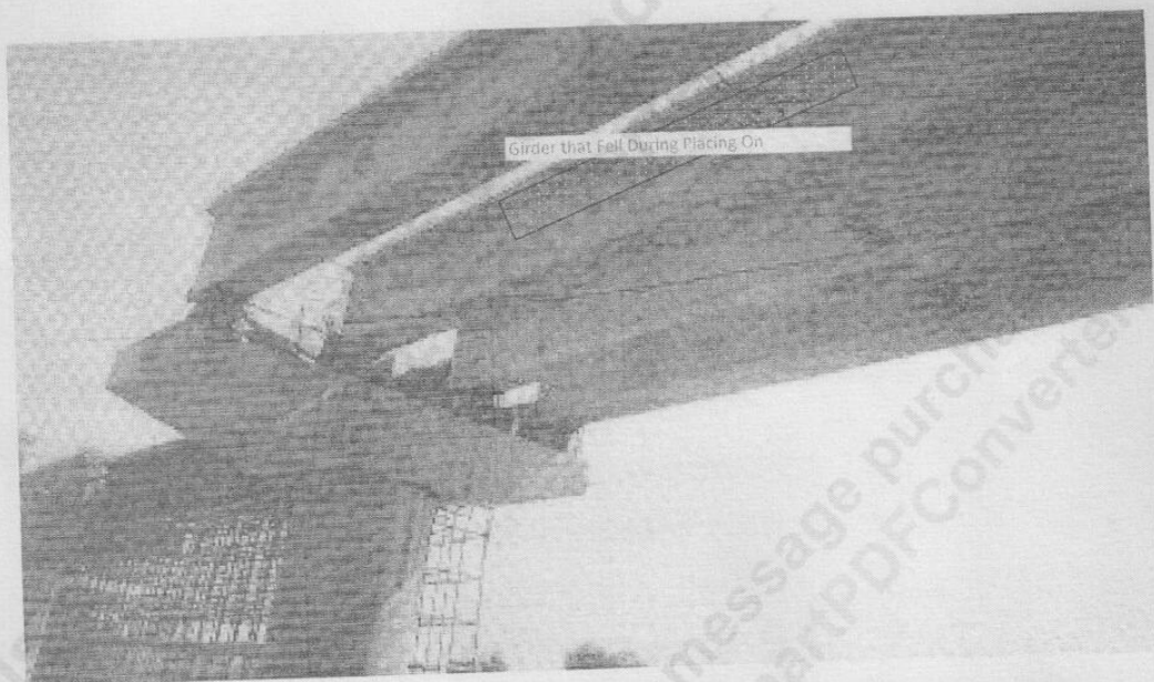
Figure 1 General View of Temporary Wooden Stand/ temporary bearing and welded metal road ( this cross-welding shall continue in future) was used to club/join all Girders in Monolithic Condition. Girders are aligned in Longitudinal Direction and Good Quality of Concrete indicated by sharp edges and N-Type Rebound Hammer reading as per IS: 13311.
